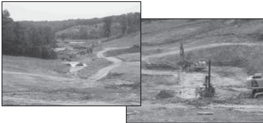
Construction has begun on the KAWC Kentucky River Pool 3 project.
