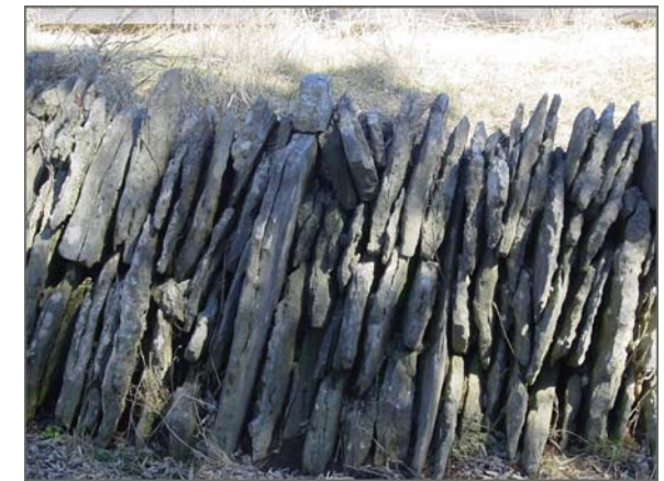
Edge fence with thin slab and wedging rocks or rocks with angled edges are inserted into the holes between the rocks.
