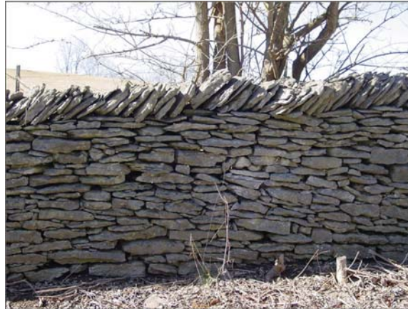
Thin course turnpike fence.
